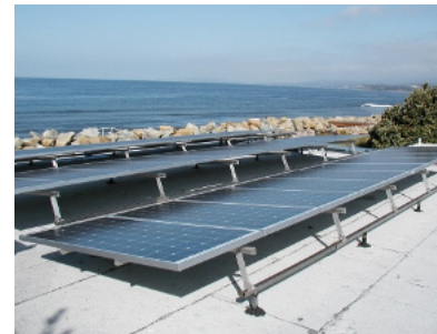
Solar panels mounted in racks
